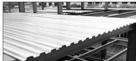
Steel deck and metal roofing
